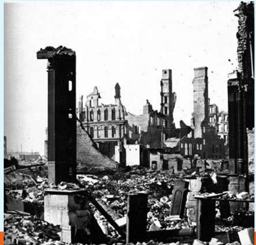
Aftermath of the fire
