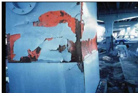
Fig. 15: Failure due to local buckling
