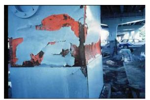
Fig. 15: Failure due to local buckling
