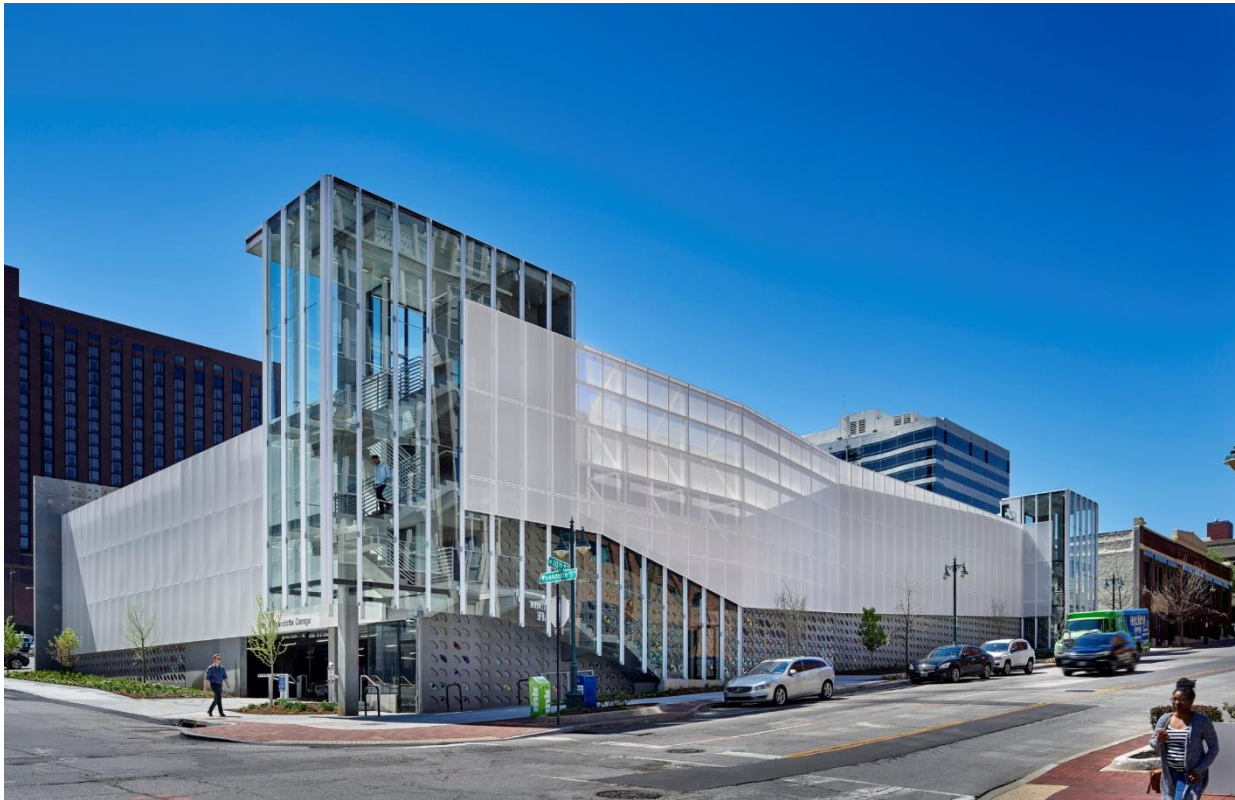
Wyandotte Parking Garage, Kansas City
