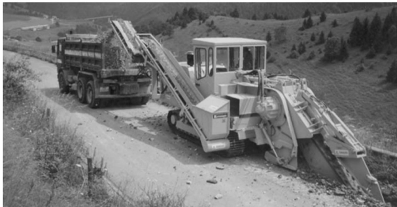
Plate 9a. A Mastenbroek 17/17 trenching machine with variable-offset heavy-duty cutting chain for trenches up to 0.6 m wide by 1.8 m depth. Larger machines are made. J. Mastenbroek & Co. Ltd, Boston, UK
