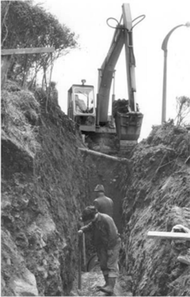
Plate 7b. An early photo showing unsafe conditions not now permissible. The designer would now have to consider any safer alternative route for the trench, or require a safe berm to be cut into the hillside first to give a shallower trench. The contractor must fully support the trench sides and require his men to wear hard hats.
