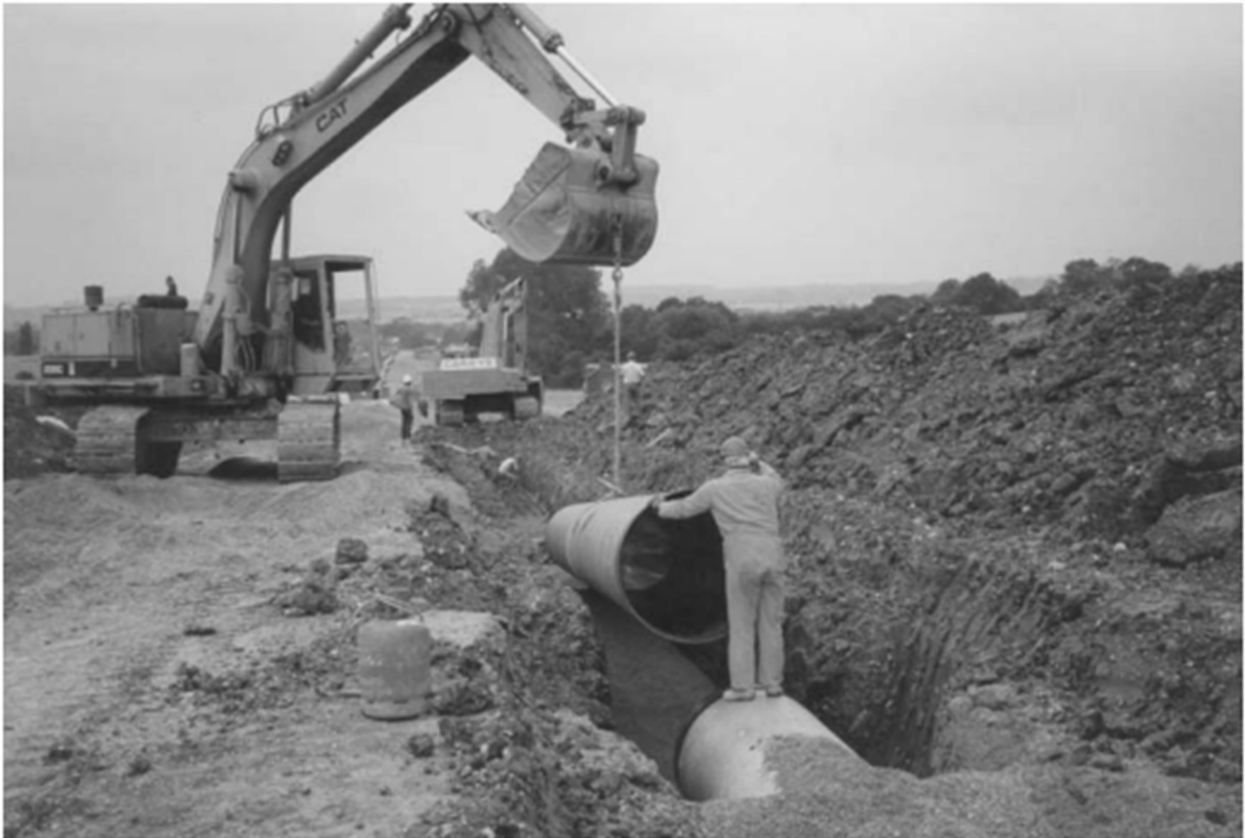
Plate 10a. It is almost universal to use the hydraulic excavator also as a crane
