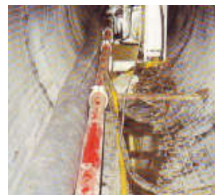
ZX delivery lines are eminently suitable for conveying muck over long distances.
