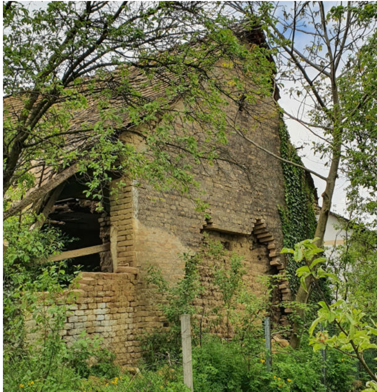
(b) Fired brick wall built to support collapsed rammed earth wall
