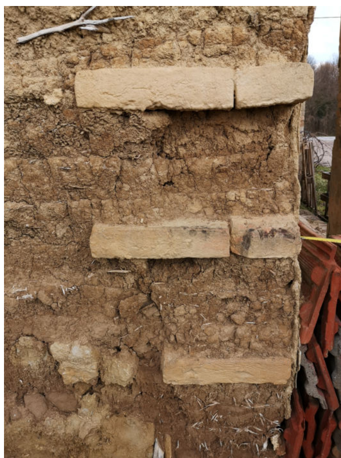
(b) A detail of corner strengthened with fired brick
