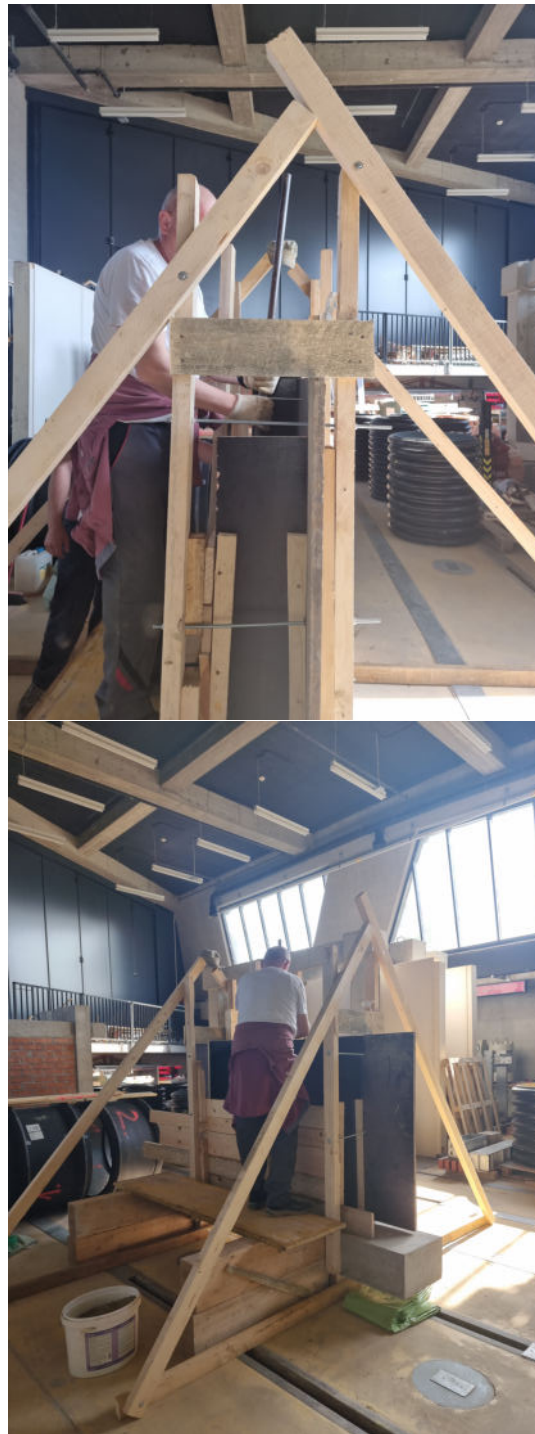
Figure 5.4: Building of rammed earth walls
