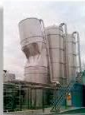
Buckling of a container
