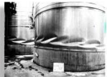
Buckling of a wine steel container, California, 1979
