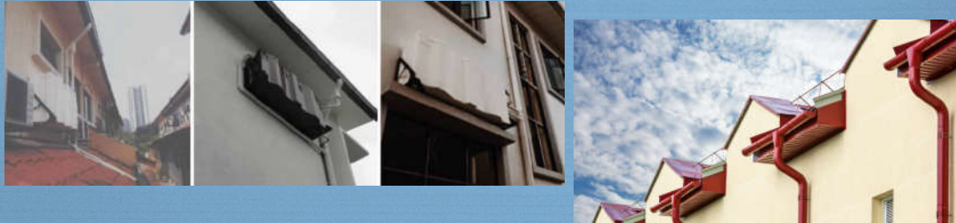
Wall – Mounted Rainwater Harwesting
